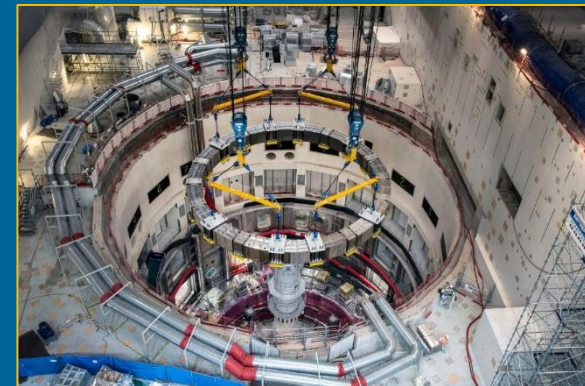
16 Sept 2021 – Poloidal field coil # 5
