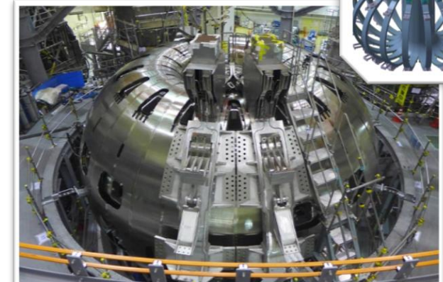
JT-60SA Toroidal Field Coil Casings
