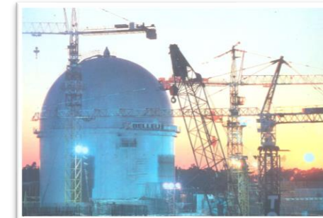
Cirene (Italy) HWR Main Steel Containment (38mm thk., ID over 33m)
